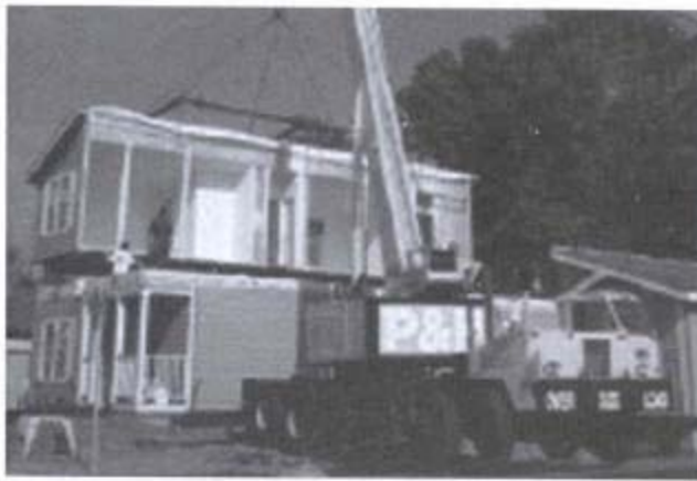
After installing the ground floor modules on the permanent foundation, the second floor modules are craned into place.
