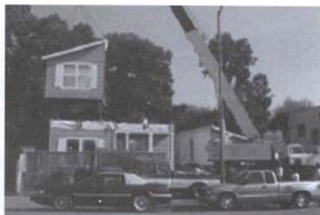
After installing the ground floor modules on the permanent foundation, the second floor modules are craned into place.
